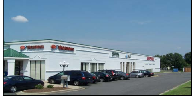
Rear View of Building (Facing I-485)
