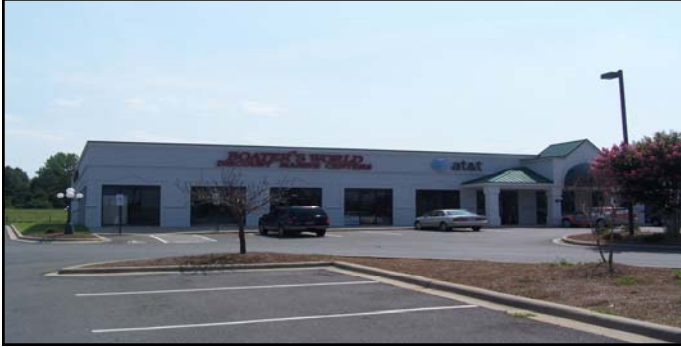
Front View of Building
