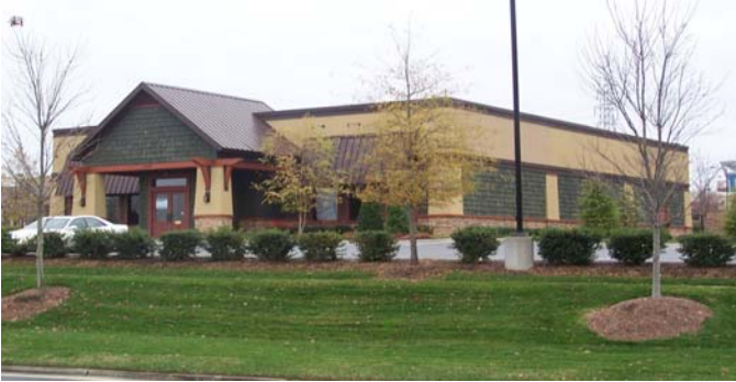
Front View of Building
